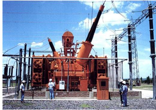
**Figure 1.** A large power transformer having long high voltage and smaller low voltage bushings mounted on top of the oil-filled transformer tank.
