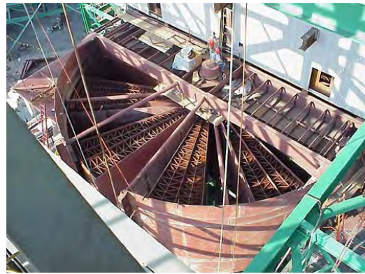
Figure 1: Typical rotary regenerative Air Preheater in phase of implementation in a coal-fired steam generators (Image courtesy of ALSTOM)
